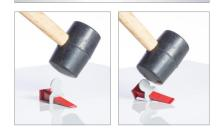
After the glue dries, break off the clips by hitting them with a rubber mallet along the gap. Only the flat foot of the clip is left under the tile, which does not interfere with the grouting, while the part of the clip with the wedge breaks off. The wedges should be gathered as they can be reused, while the remains of the clips should be discarded. **HIGHLIGHTS**
