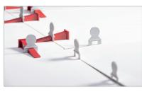
Lay further tiles on the clips, adding further clips under the outer edges. A gap thicker than 1 mm can be obtained by using cross-shaped spacers of the appropriate thickness.
